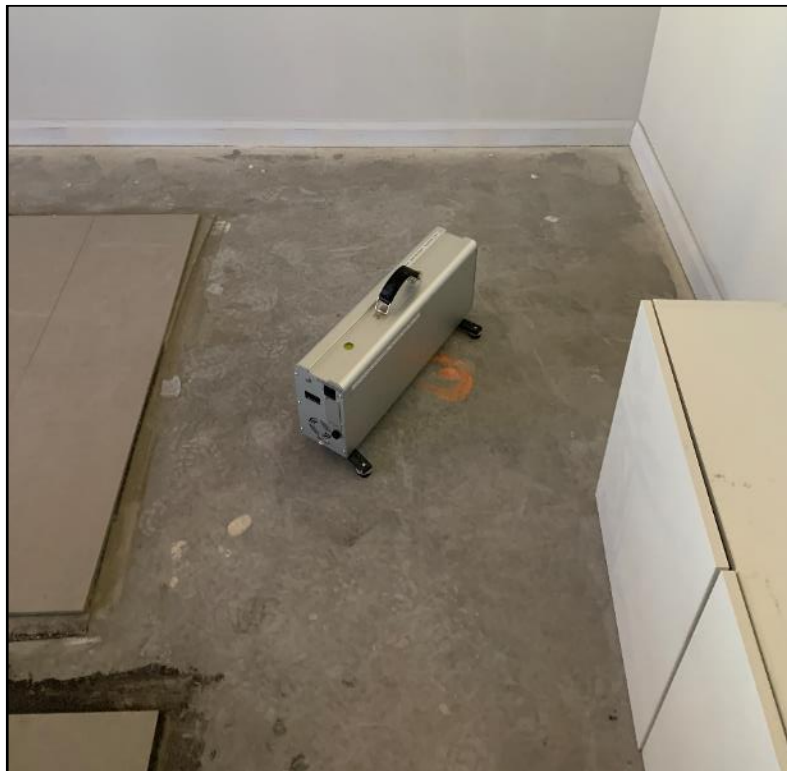
Figure 3. Source room & test 3 floor (bare concrete slab)
